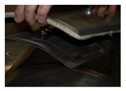
**Step #3** Pull access door outward insuring the centering stops of door interior are securely fitted into duct opening, centering door. Tighten wingnuts by hand one at a time until door is stable in centered position, then torque to 30 inch pounds.
