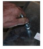
Loosen both wing nuts to separate door halves enough to slip access door into duct opening being careful not to damage gasketing.
