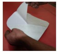
Remove the protective backing from the template supplied with the respective sized access door and center on the duct, in the appropriate place; provide a minimum 2" from any edge of the duct. When the grease duct passes through a partition or wall, maintain combustible clearance as per Grease Duct Manufacturer requirement.
