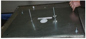
Step #3 Pull access door outward insuring the centering stops of door interior are securely fitted into duct opening, centering door. Tighten wingnuts by hand one at a time until door is stable in centered position, then torque to 30 inch pounds.
