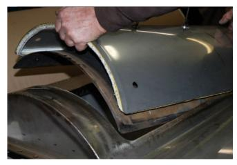
Step #3 Pull access door outward insuring the centering stops of door interior are securely fitted into duct opening, centering door. Tighten wingnuts by hand one at a time until door is stable in centered position, then torque to 30 inch pounds.
