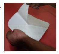
Remove the protective backing from the template supplied with the respective sized access door and center on the duct, in the appropriate place; provide a minimum 2" from any edge of the duct. When the grease duct passes through a partition or wall, maintain combustible clearance as per Grease Duct Manufacturer requirement.
