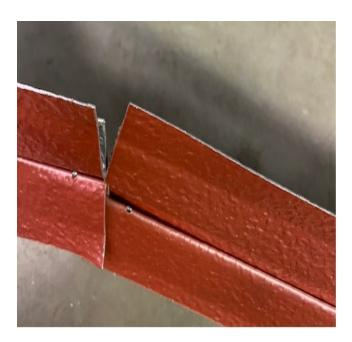
4) Fully seat the small end of one Zed Rib 2" into the large end of the next Zed Rib as illustrated in succession until the full length of Zed Rib between horizontally running Zed Rib and the starter and/or finish cap.
