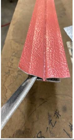
**3)** Then slip the small end of one telescopic Zed Rib into the large end of the next telescopic Zed Rib.
